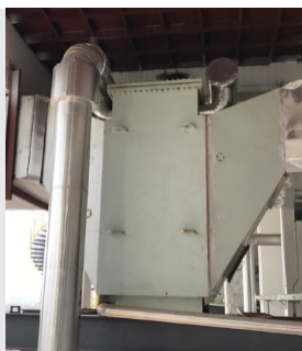
Indirect contact type (Suitable for 100t gas boiler) (2.8m*3.6m*3.45m)
