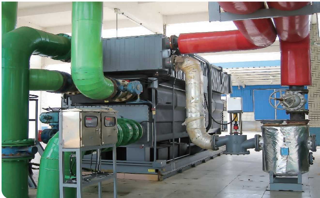
Triple Generation Hot Water Chiller
