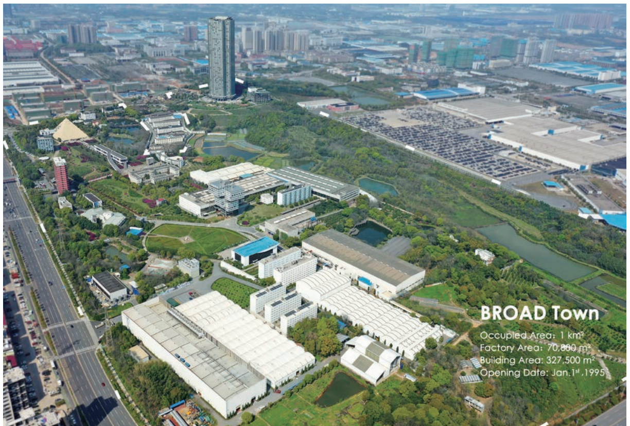
BROAD Town — BROAD central air conditioning R&D and production base (Changsha, Hunan)
