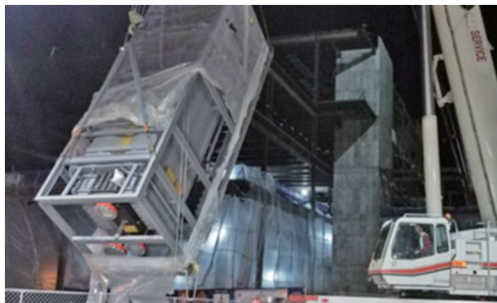
Onsite Rigging 吊装现场
