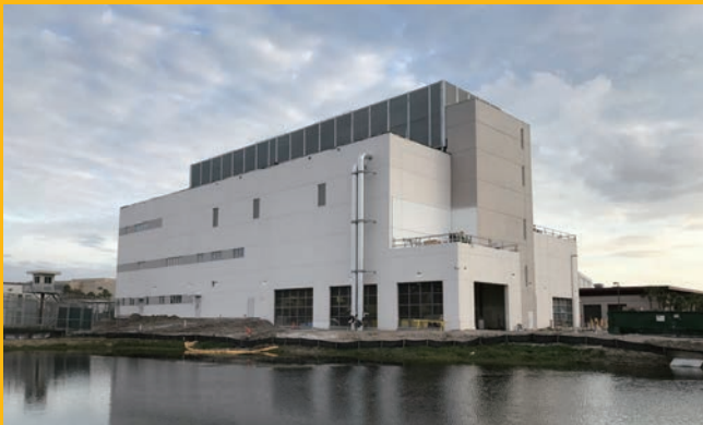
Pinellas County Jail Infrastructure Building 皮涅拉斯县监狱基础设施楼
