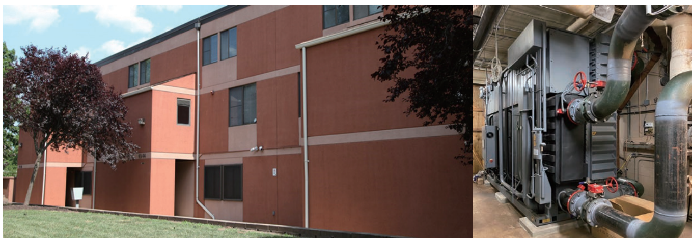
Marvin Apartments & Mechanical Room 马文公寓及机房
